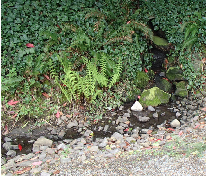
Photo No. 12 Looking east at pipe end discharging to roadside swale just upstream of inlet pipe upstream of CB #30a-38 at House #6065. Swale appears stable with small rock riprap and other cobbles. It appears some of the flow may be diverted south at CBa-37 (see Photo #11) to reduce impacts to this open swale.
