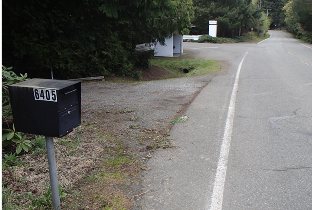
Photo No. 1 Standing adjacent to the site and looking north at the open ditch on the West side of West Mercer Way (toward CB 30a-26)
