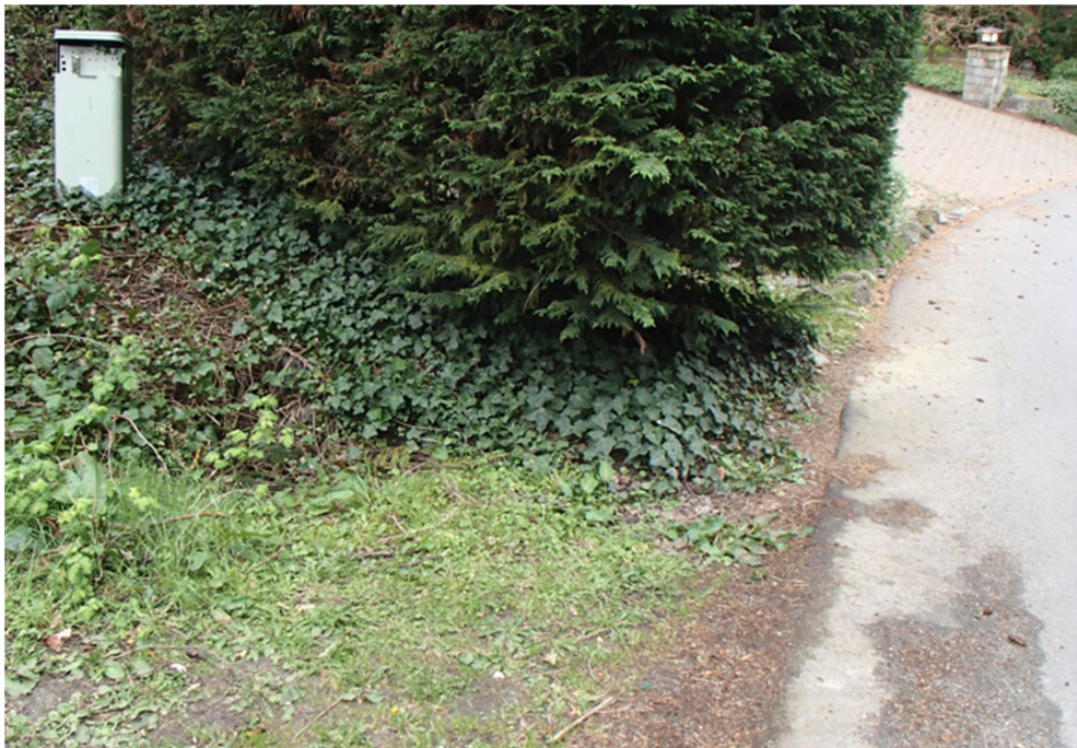
Photo No. 11 Looking southerly at CB #30a-37 just south of House #7820. Note ivy overgrowth but CB appears to be draining. Minor indication of erosion at the pavement edge. Inlet in street appears to be full of sediment (CB#30a-43) not on main line, so no impact to conveyance capacity.
