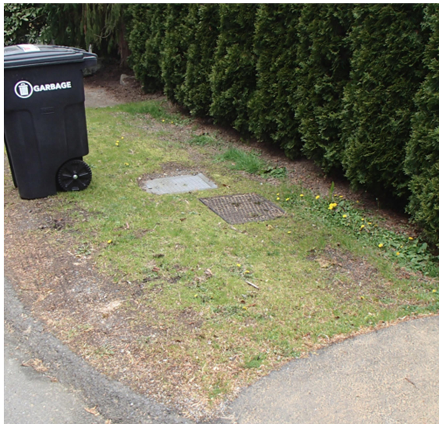
Photo No. 6 Looking northwesterly at CB 30a-25 (solid cover) where the SD crosses to the south side of the street and connects to CB 30a-34.
