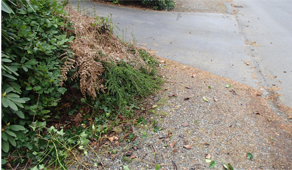
Photo No. 9 Looking southerly at CB #30a-17 adjacent House #6030. Note ivy growing over grate, but it appears to be draining and not signs of surface bypass flow. Photo is past end of ¼ mile Downstream Analysis. Further review downstream completed to confirm outfall to Lake Washington.
