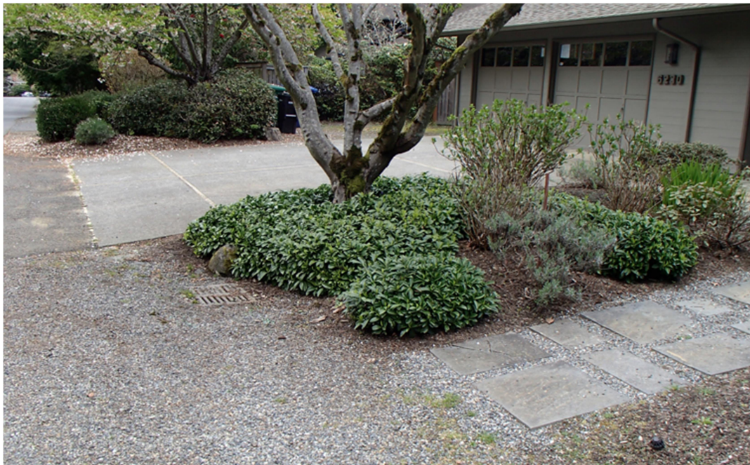
Photo No. 2 Standing on the east side of 79 th Ave. SE, looking north at CB 30a-7 in front of House #6320
