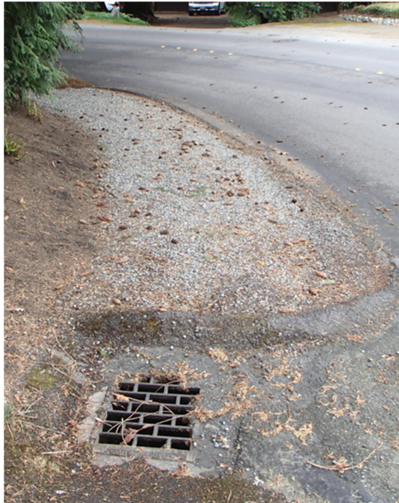
Photo No. 7 Looking southwesterly at CB30a-52 opposite House #6019 and #6017. Note gravel lip and vaned grate to catch runoff down steep road grade.
